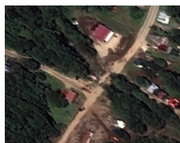
After: DigitalGlobe FirstLook imagery clearly shows damaged areas
